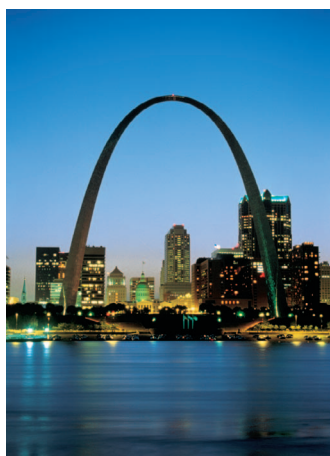
Glen Allison/Stone/Getty Images The design of the Gateway Arch in St. Louis is based on an inverted hyperbolic cosine curve (Exercise 73).
